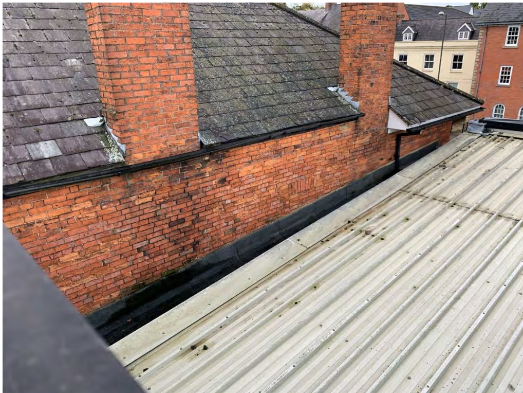
Plate 4: Exposed Northern elevation
