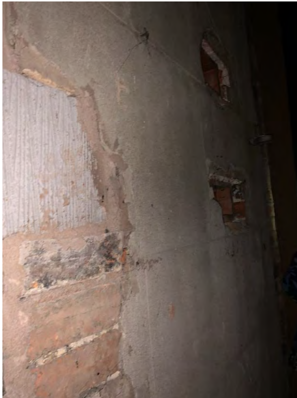
Plate 5: Potential fragment of original render on rear elevation
