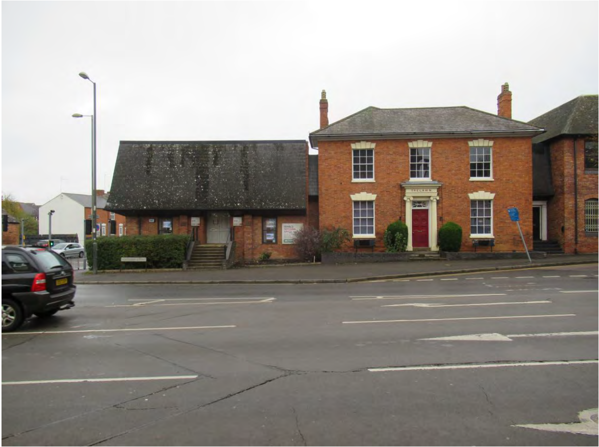
Plate 1: Trelawn Grade II Listed Building and adjoining later buildings
