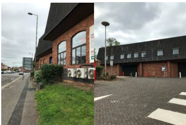
Photograph 1 and 2: Eastern aspect of building and ornamental planting and amenity grassland on northern aspect.
