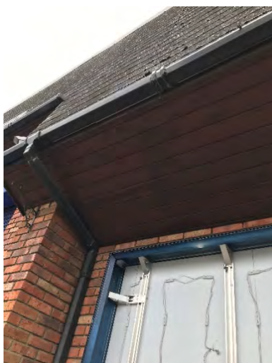
Photograph 3: Eastern aspect of building showing wooden soffits.
