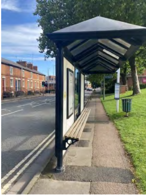
Photograph 16: Bus Stop Seated Area
