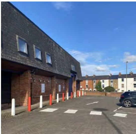
Photograph 3: Existing Site Conditions (Western)
