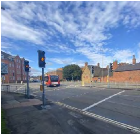
Photograph 9: Signalised Pedestrian crossing (northwest along Castle Street)
