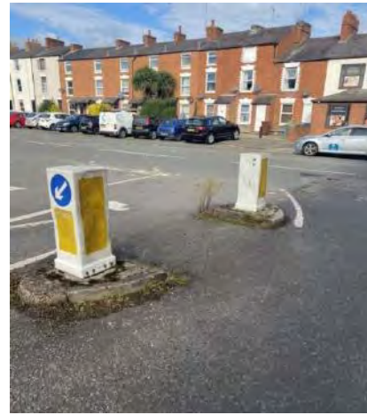
Photograph 10: Pedestrian Refuge Island on Bolton Road/Castle Street Junction
