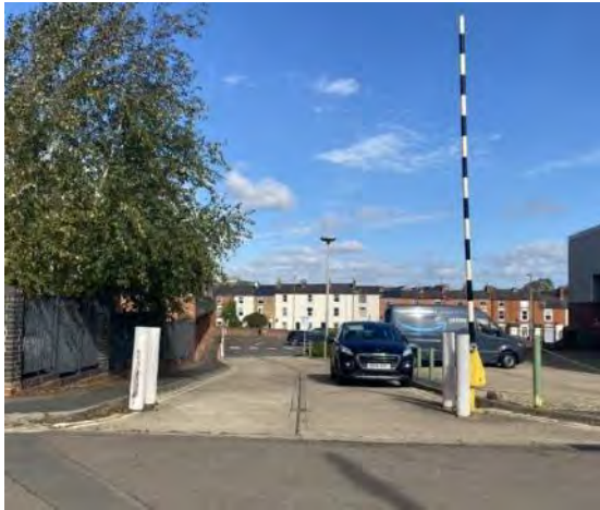
Photograph 1: Existing Site Access
