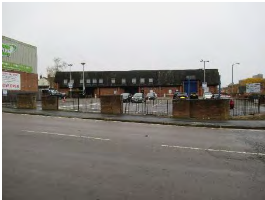
Plate 1: View towards the Site from Bolton Road
