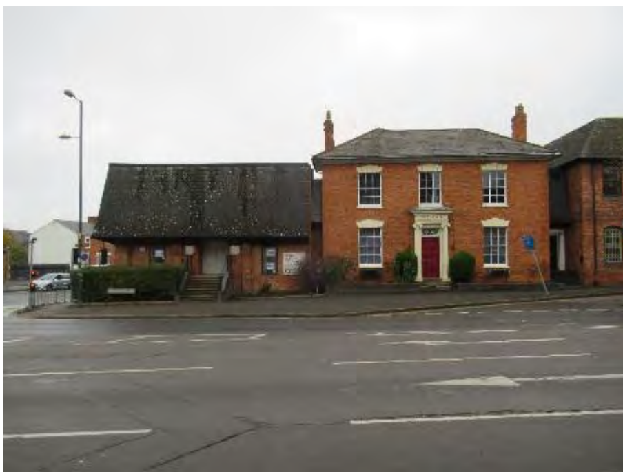
Plate 4: View towards Trelawn from the west
