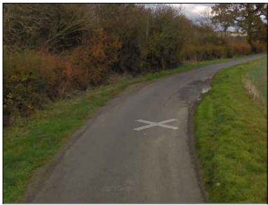
Informal Passing Place on bend Road width = 2.9m approx
