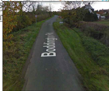
Informal Passing Place Road width = 3m approx Vehicle tyre tracks indicate use
