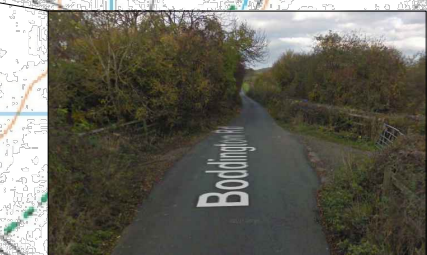
Informal Passing Place at field access Road width = 3m approx
