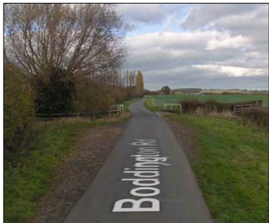
Informal Passing Place at canal feeder Road width = 3m approx
