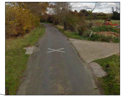
Barn access used as passing place - worn down verge Road width = 3m approx
