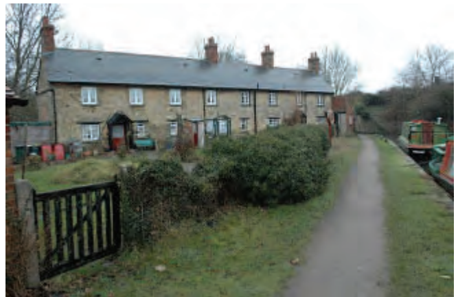
Cottages at Kidlington Wharf: former warehouses
