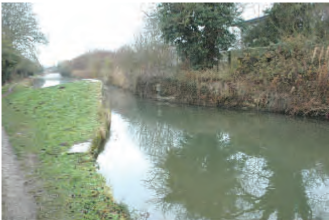
Pillbox and bridge abutments
