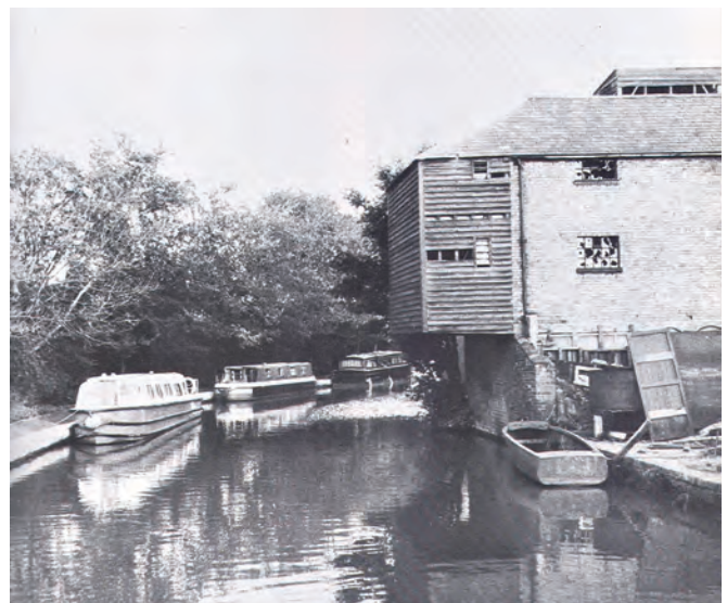
The Paving & Lighting Commission stoneyard building established in 1825 seen in 1974 (Trinder 1982)
