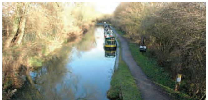
View north from March Bridge to the moorings
