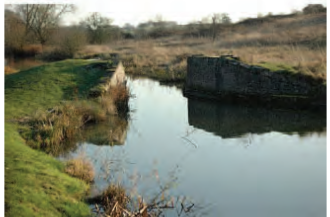
Abutments of former bridge 169
