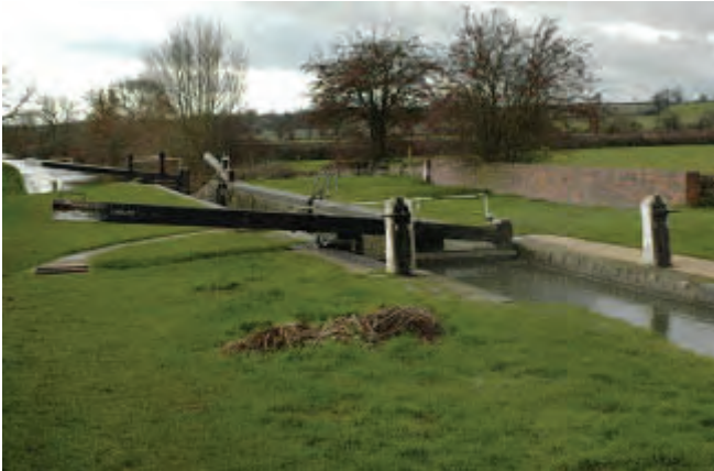
Slat Mill Lock set in an expanse of fields
