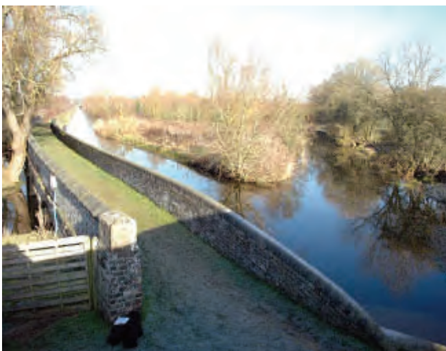
Cherwell Crossing over Aynho Weir Lock south of Nell's Bridge
