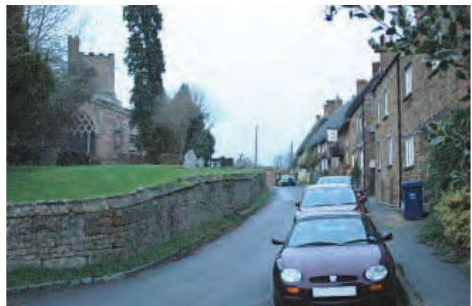
The view west from bridge 152 up Red Lion Street, past the Church and Red Lion Inn
