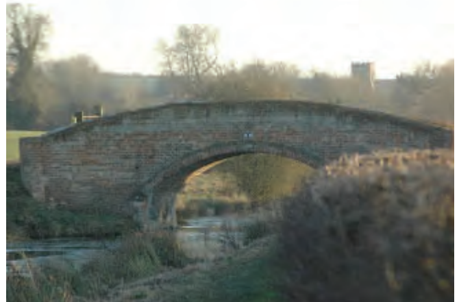
Bridge 202 with Upper Heyford church tower visible in the distance
