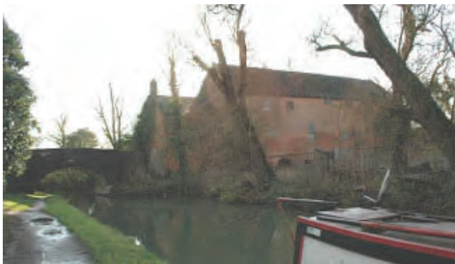
Bourton Mill and adjacent bridge
