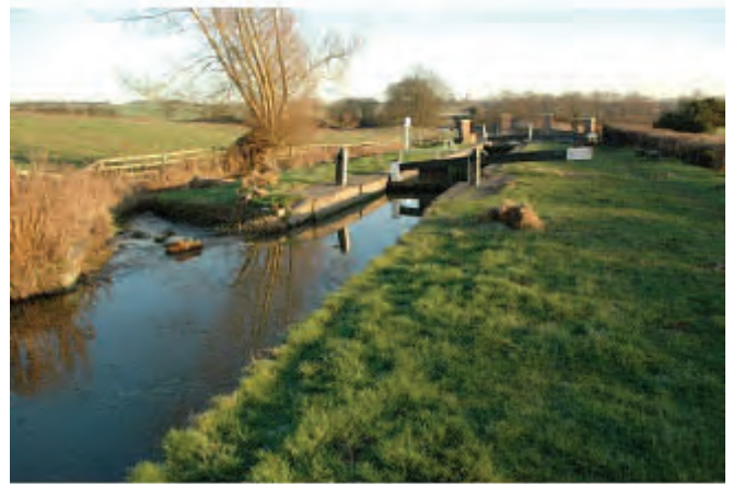
Somerton Deep Lock
