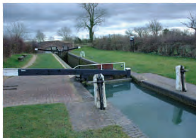
Claydon Middle Lock, typical of those north of Banbury, with double gates at the tail
