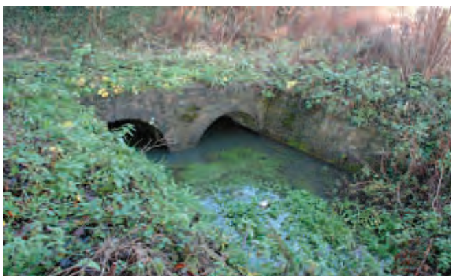
Double arched culvert under the canal at the southern end of a shallow embankment near Clattercote
