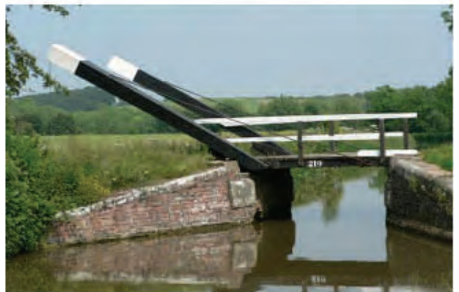
Shipton lift bridge in the closed position
