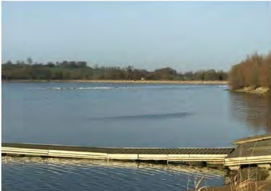
11 th December 2018: Photo of northern half of reservoir showing water level not recovered and shallows in middle evidenced by birds standing.
