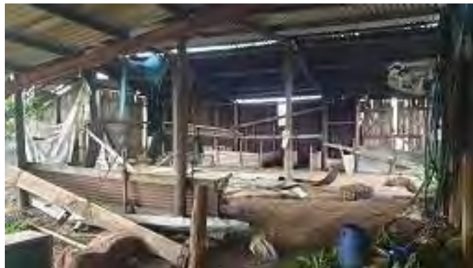
Figure 2 – timber lean-to which will be demolished
