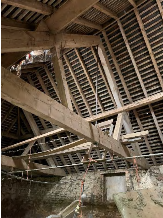
Figure 14: Views of building 4 – top, the rear (west) elevation showing ironstone ashlar construction but with some rebuilding in brick; bottom left, the late 19 th /early 20 th -century roof trusses and modern roof covering over them; bottom right, the date 1962 in the concrete floor. Vegetation is engulfing this elevation – compare with Soden 2016, figure 9.
