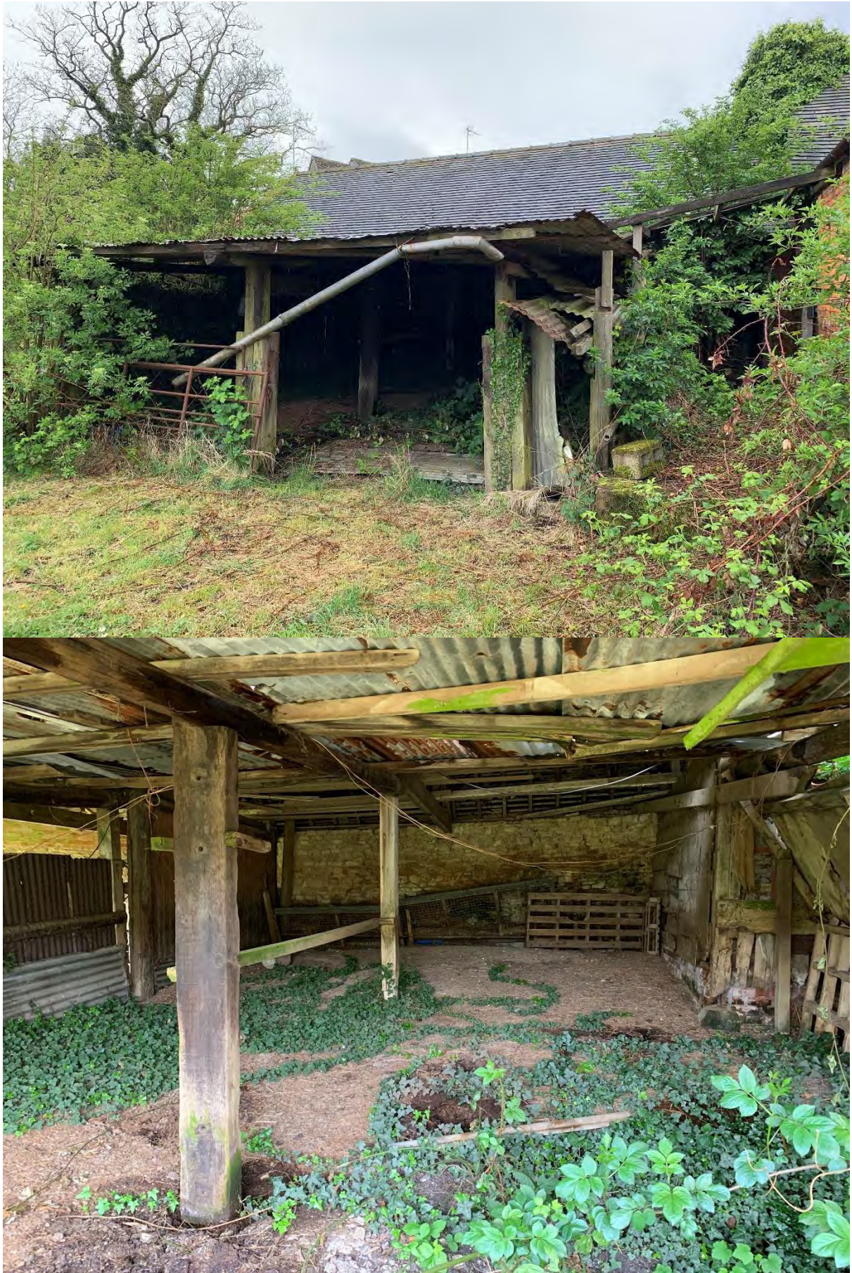
Figure 15: Views of the 'ramshackle' extension, building 3, in front (north) of building 2.
