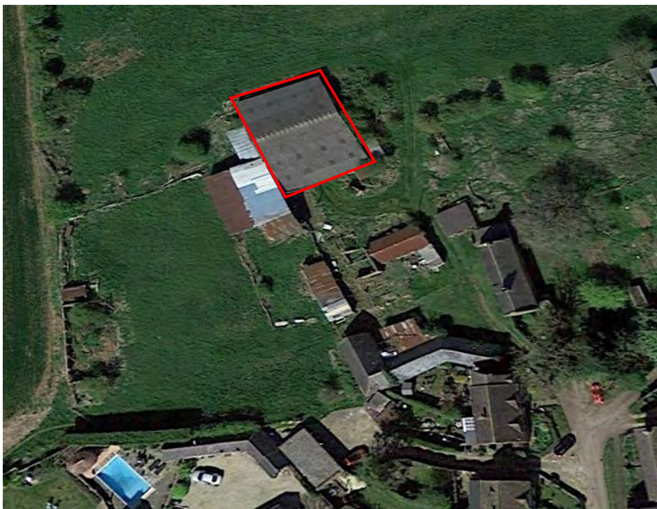
Figure 3 – Aerial image from 2017 (Source: Google Earth)
