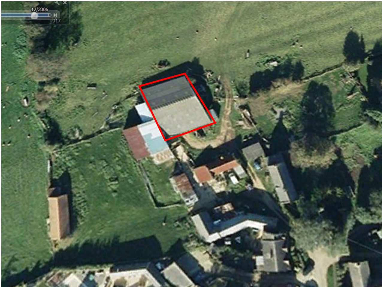
Figure 1 – Aerial image from December 2006 (Source: Google Earth Pro)
