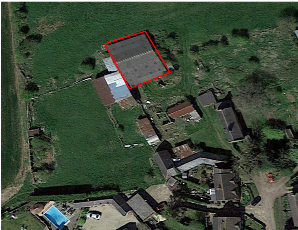
Figure 3 – Aerial image from 2017 (Source: Google Earth)
