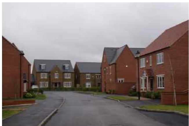
Image 2: Local ironstone (or a modern day equivalent) units terminating the views. An example of the larger / key plots which are responding to local vernacular
