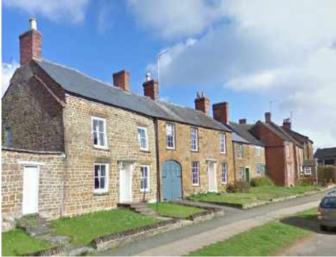
A short terraced run of properties on High Street. Variations in ridge and eaves line adds interest to the street scene.
