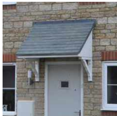
Unsuccessful example of plastic faux-tile porch, Banbury
