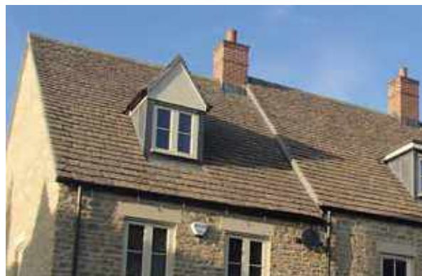
Good examples of modern dormer windows, pitched roofs, slate tiles and brick chimneys, Woodstock
