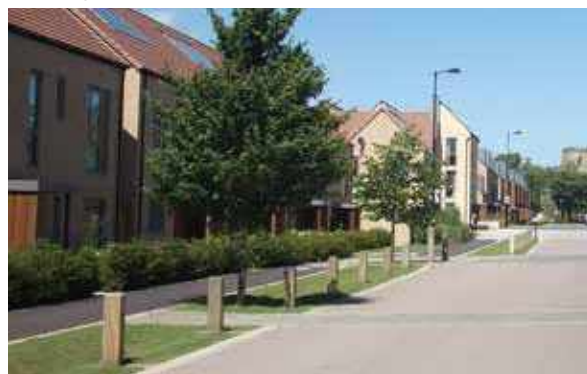
Incorporating SuDS along kerbside, Trumpington Meadows, Cambridge
