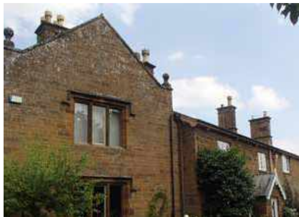
Two to three storey buildings, Adderbury
