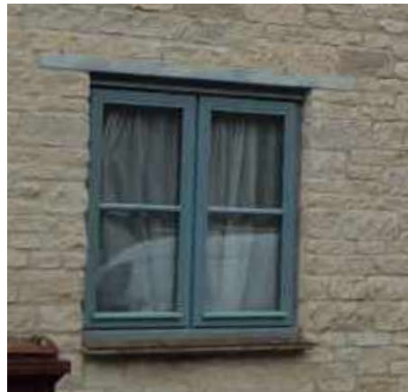
Casement window flush with wall, Bletchingdon
