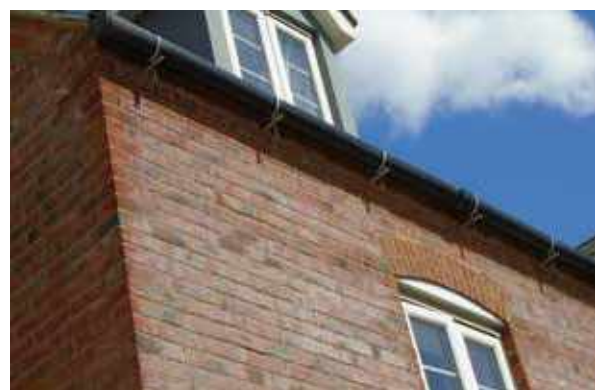
Guttering, South West Bicester
