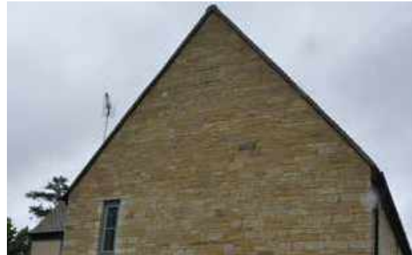
Steeply pitched roof with no overhang, Bletchington
