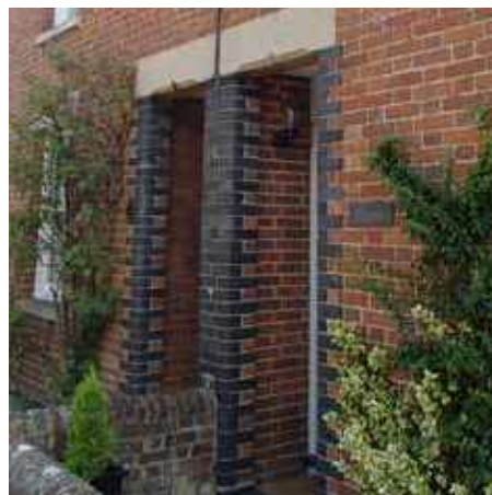
Localised brick detail around doorways
