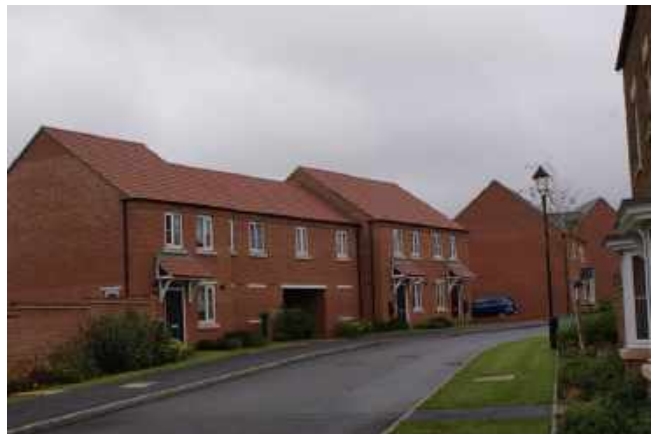
Image 1: Terraced brick units with rear courtyard access
