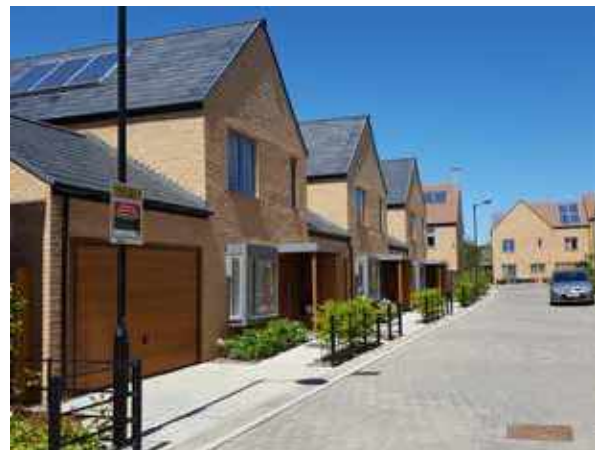
Photovoltaic panels, Trumpington Meadows, Cambridge
