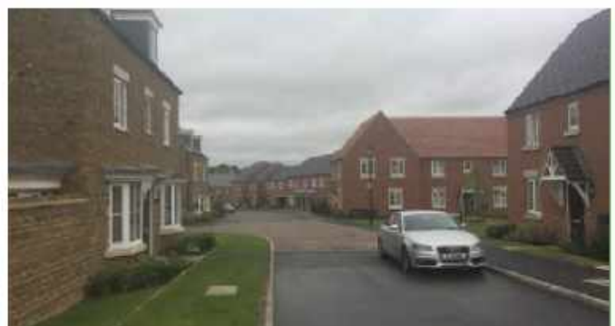
Example of new dwellings in the south-west of Adderbury
