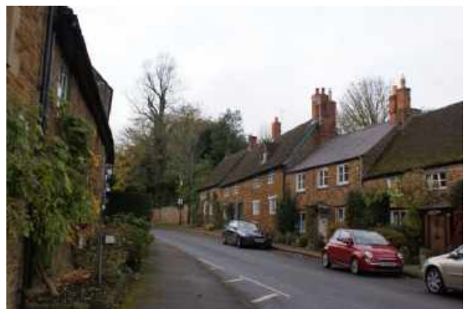
Traditional terraced properties along Cross Hill Road
