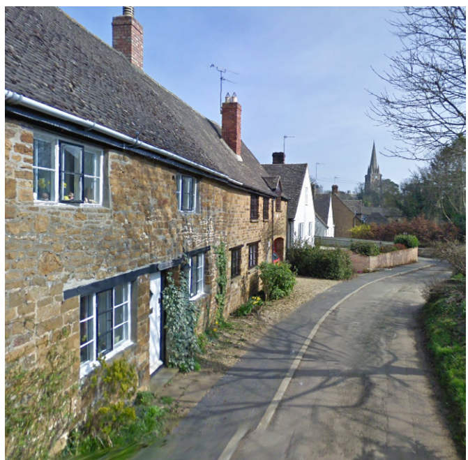
Strong enclosure to the street framing view towards The Church of St Mary
