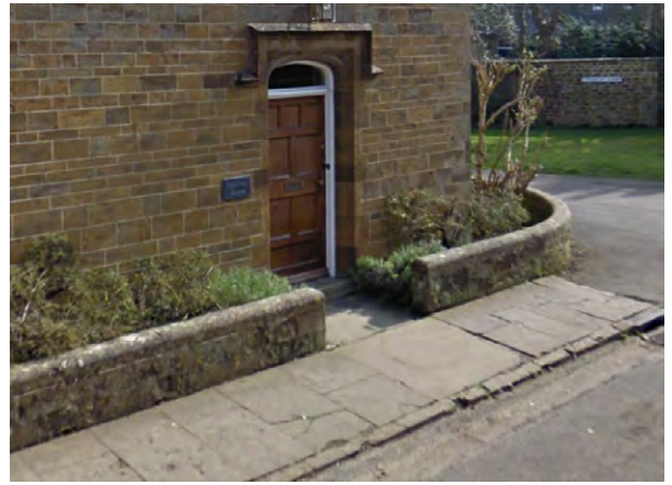
Low stone wall boundary on Mill Lane
