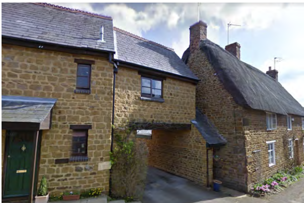
Undercroft through to parking court
