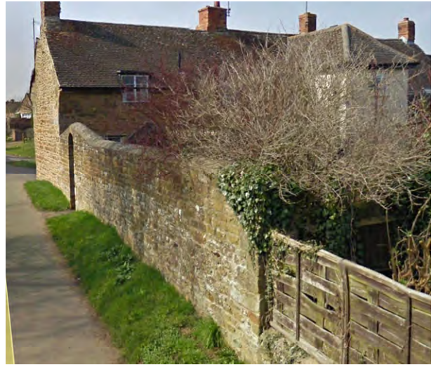
High stone wall boundary facing public realm
