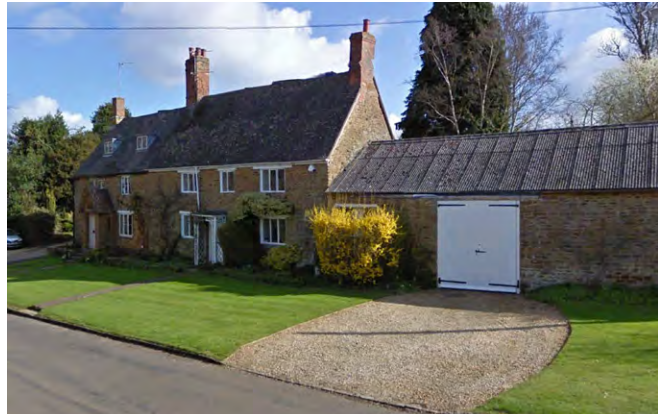
Simple front gardens, wide fronted properties and linked garages - Horn hill Road
