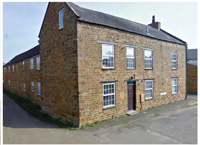
This key corner unit has an enhanced floor-ceiling height when compared to the nearby properties.
