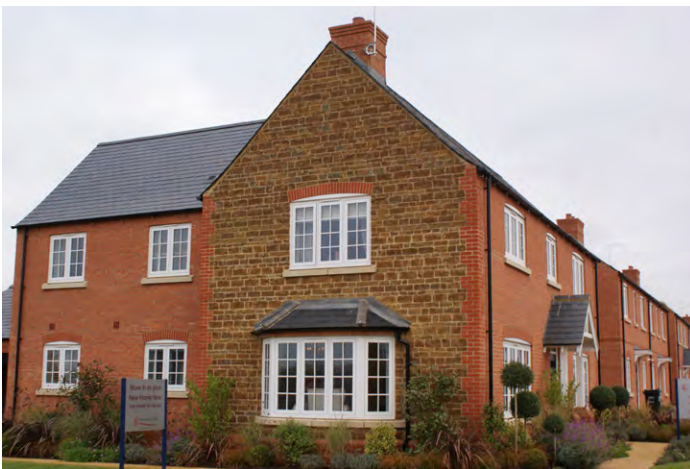
An example of a key corner unit utilising a change in material and a bay window on the most prominent facade
