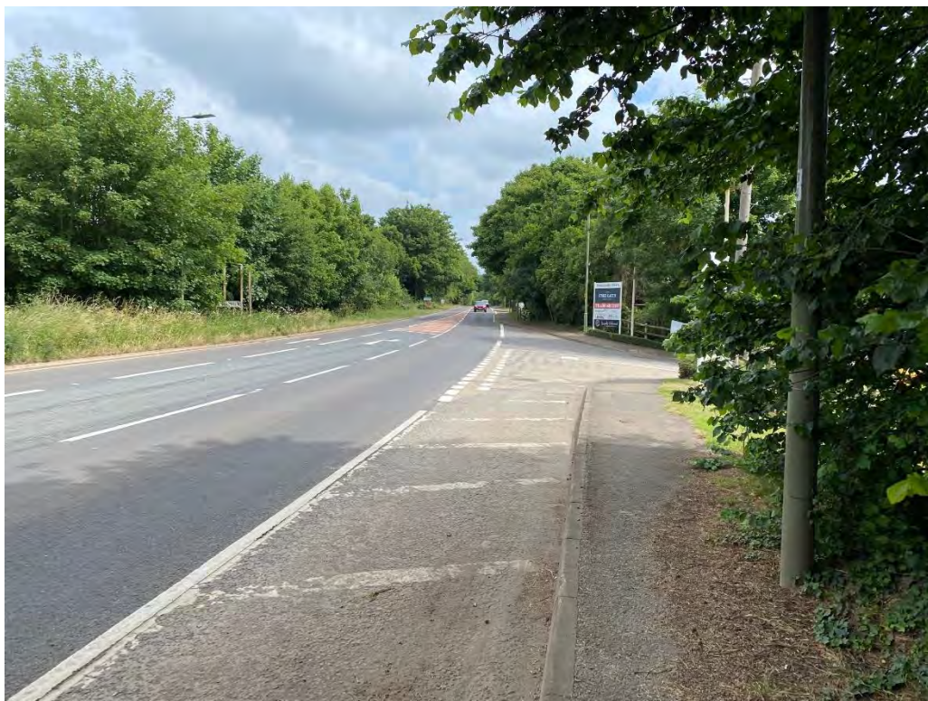
Photograph 1 – A section of the walking route along Oxford Road to Adderbury Day Nursery
