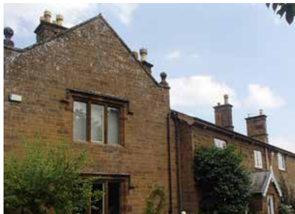
Two to three storey buildings, Adderbury
