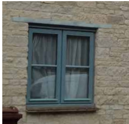
Casement window flush with wall, Bletchingdon
