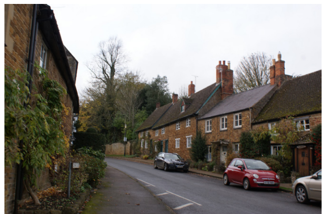
Traditional terraced properties along Cross Hill Road
