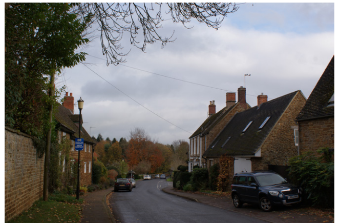
Traditional terraced properties along Cross Hill Road
