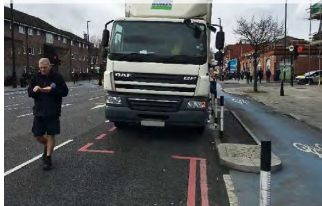
Figure 6.18: Local kerbed island for servicing across light segregation facility
