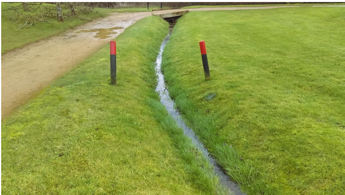
Photograph 1 : Ditch in January 2019.
