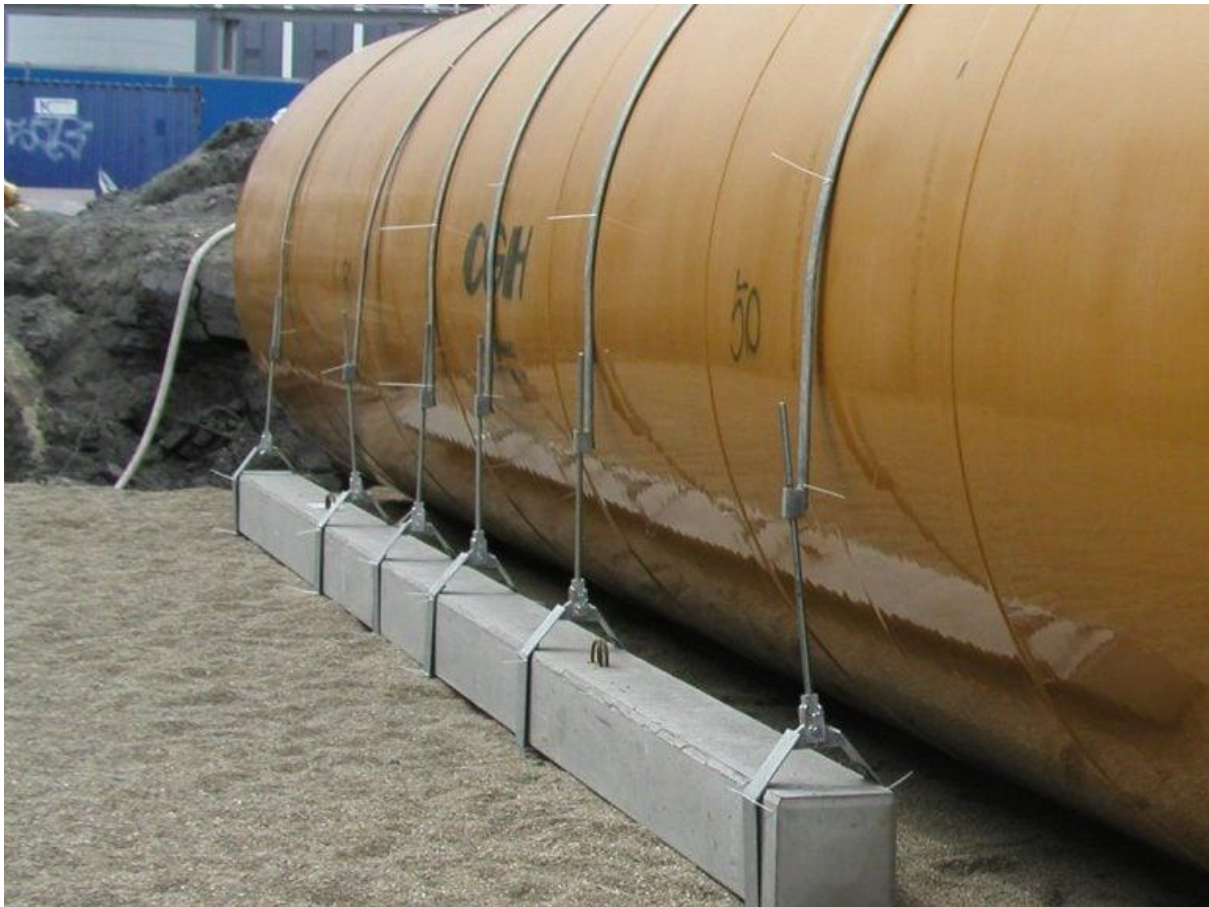
Image of GRP tank held down with concrete beam and anchoring tanks
