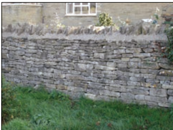
Figure 39: Chesterton Lodge boundary wall.
