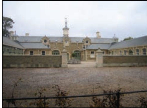
Figure 11: South Elevation of Chesterton Court, former stable block.
