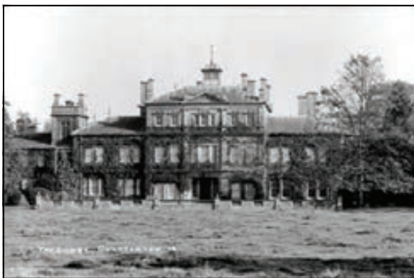
Figure 10: Chesterton Lodge as seen in the early part of the 20th Century.
