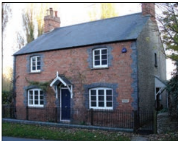
Figure 19: Hill Side Cottage
