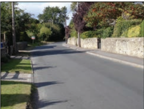
Figure 33 Main road surface
