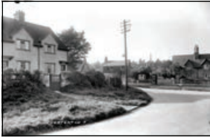
Junction of Green Lane and Alchester Road.
