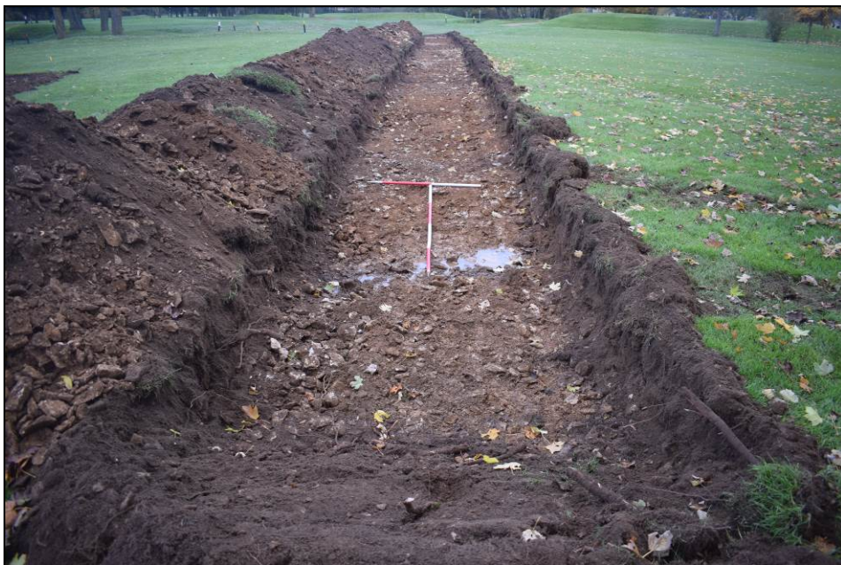
Plate 20: Post excavation of Trench 10
