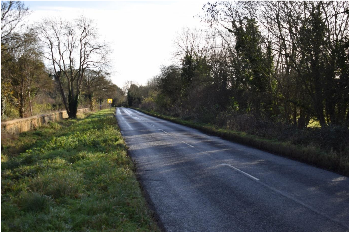
Photo 13 From A4095 looking south east in vicinity of entrance. Site on right. Bignell Park to left. Verges lost by road widening & shared footway /cycleway. Kerbs, white lining & signs introduced.
