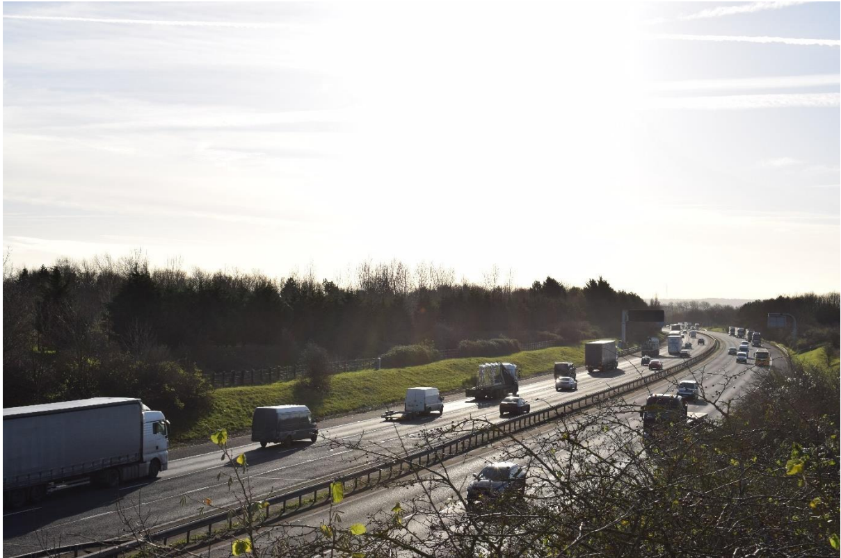
Photo 11 From A4095 bridge over M40 looking south east to site.
