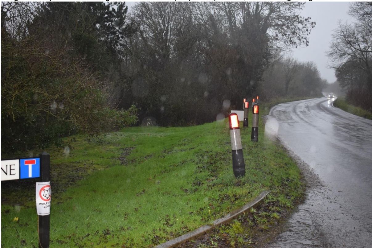
Photo 14 From A4095 looking north west showing change of levels where diverted PROW will join 2.5m wide shared footway / cycleway. Note level change and vegetation in verge.
