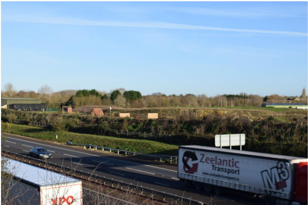
Photo 8 From Green Lane bridge over M40 looking north to site.
