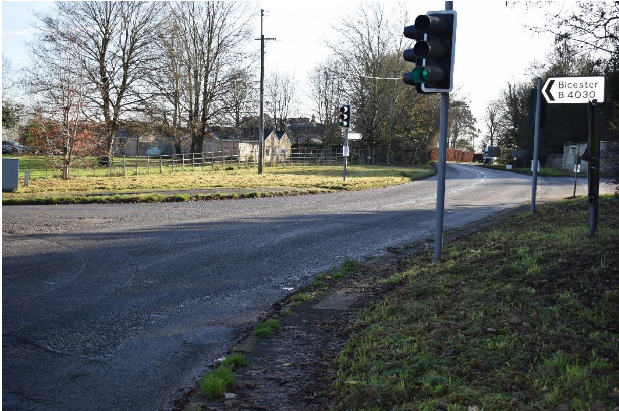
Photo 21 Middleton Stoney. Verge removed to right for footway and road widened in left verge
