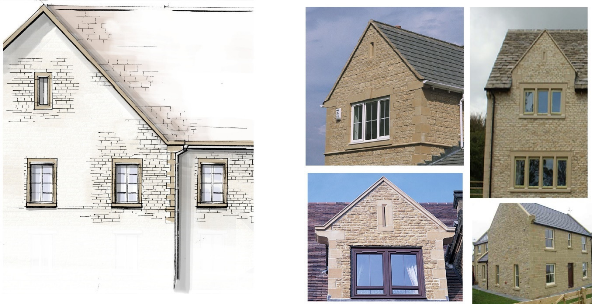
Figure 11: Examples of windows used in EPR's design that directly reference the fine stone detailing of the local area. Taken from page 36 of the DAS
