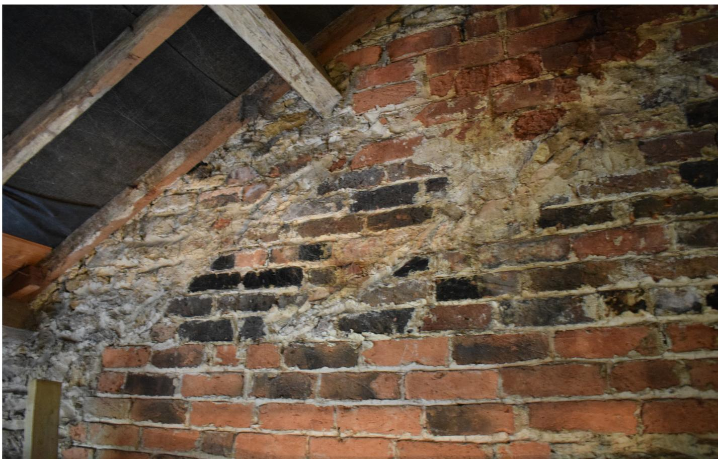
The partition wall to the service range, showing the chimney stack (removed on the ground floor) and the realigned and widened roof span.
