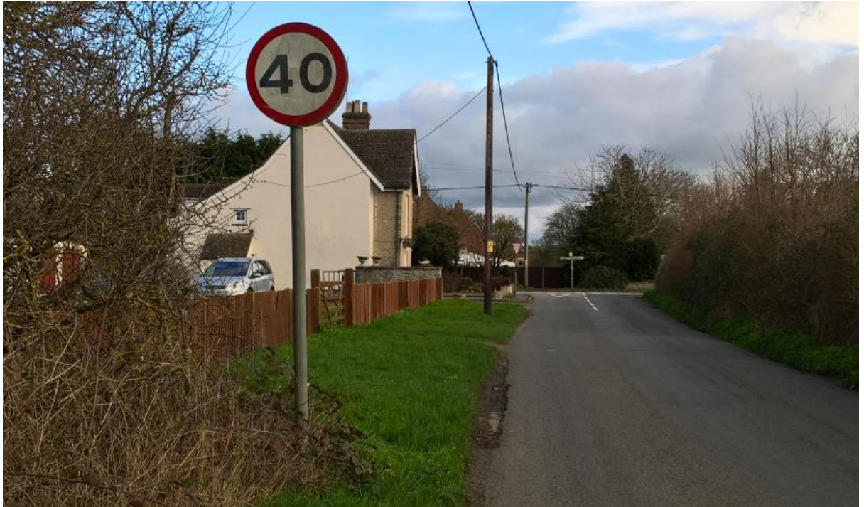
Fig. 3 Looking south-east along Aunt Ems Lane, with the site to the left
