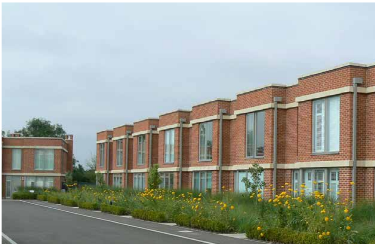
Consistent street frontage, Bicester
