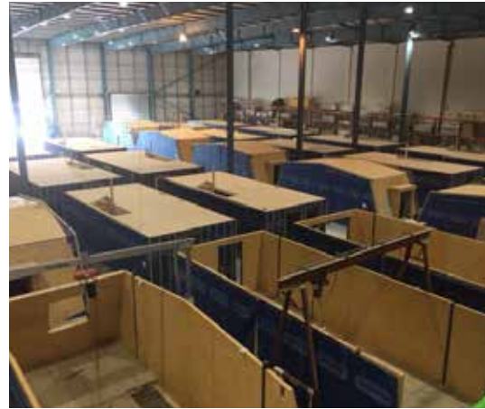
Modular construction factory, Ashford (image courtesy of Brooke Homes)
