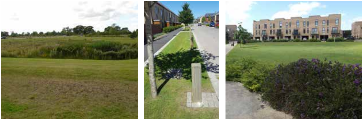
From left: attenuation pond, South West Bicester; swale, Trumpington Meadows, Cambridge; dry detention basin within parkland, Clay Farm, Cambridge.
