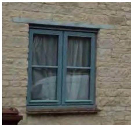
Casement window flush with wall, Bletchington
