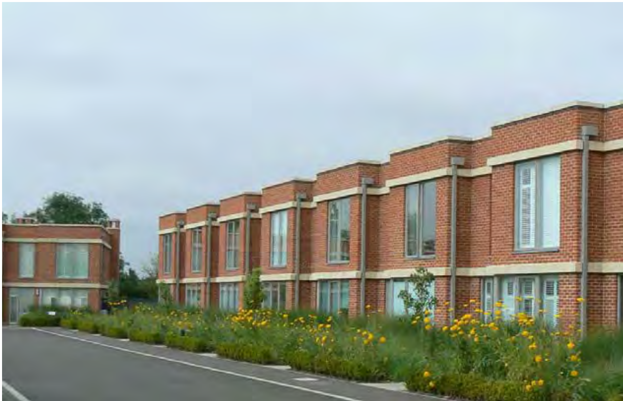
Consistent street frontage, Bicester
