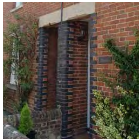
Localised brick detail around doorways
