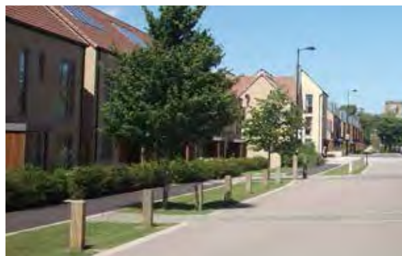
Incorporating SuDS along kerbside, Trumpington Meadows, Cambridge
