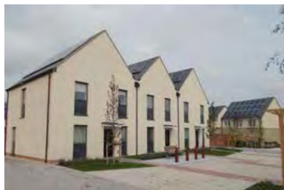
A shared surface street - NW Bicester
