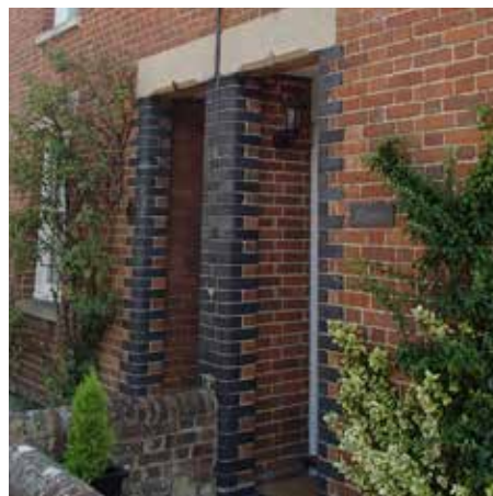
Localised brick detail around doorways
