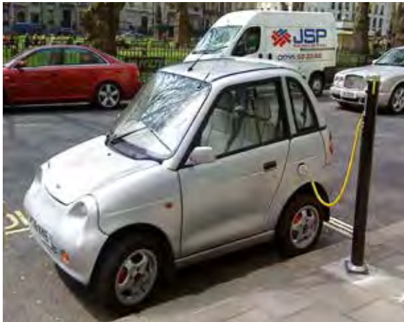
Electric vehicle charging point.
