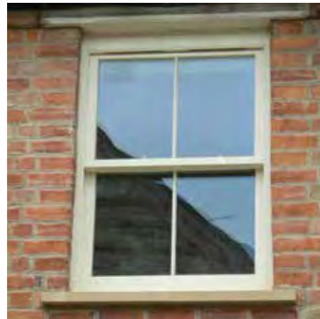
Sash window, Woodstock
