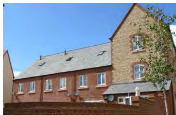
Small rooflights on rear elevation, South West Bicester
