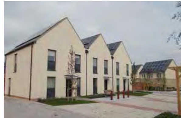
A shared surface street - NW Bicester
