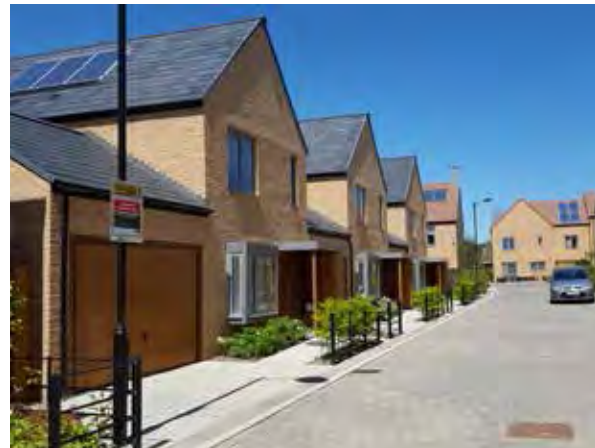
Photovoltaic panels, Trumpington Meadows, Cambridge
