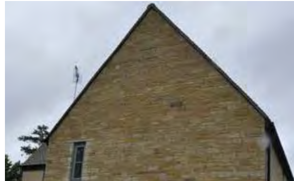
Steeply pitched roof with no overhang, Bletchington
