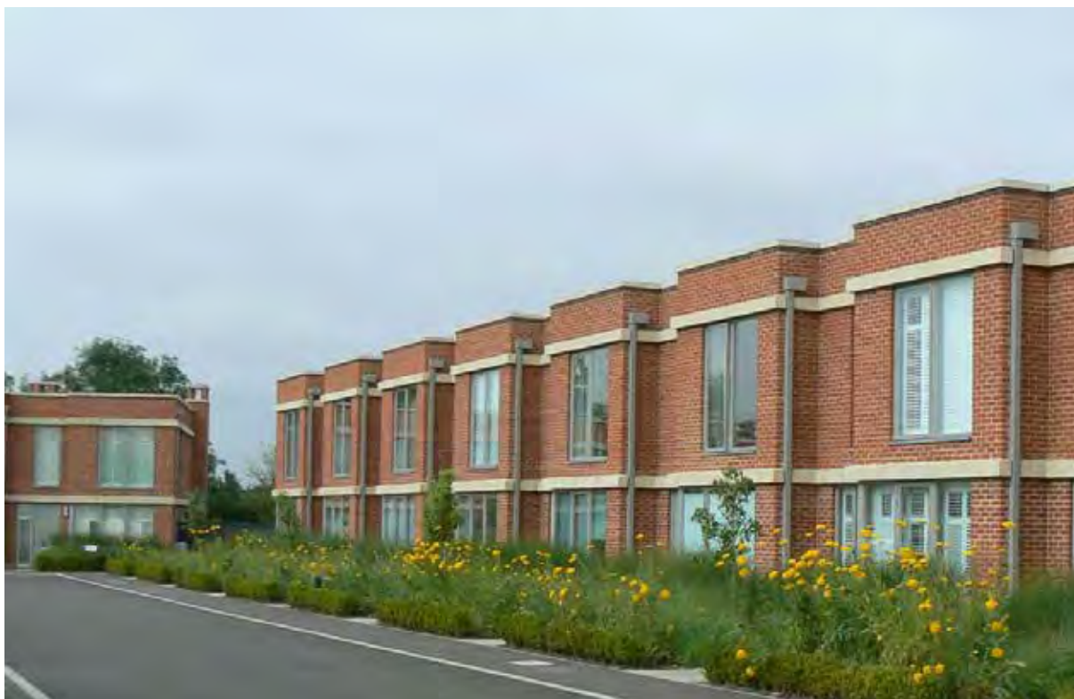
Consistent street frontage, Bicester
