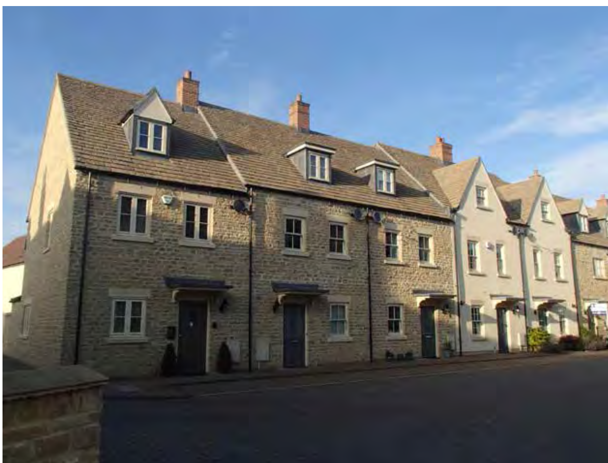
The use of locally appropriate, high quality materials must be considered early on - Ashford Close, Woodstock
