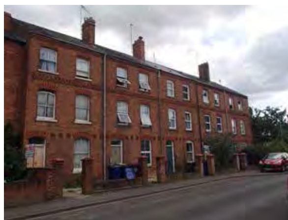
Narrow fronted 3 storey terrace, Banbury
