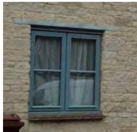
Casement window flush with wall, Bletchingdon
