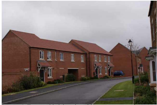
Image 1: Terraced brick units with rear courtyard access
