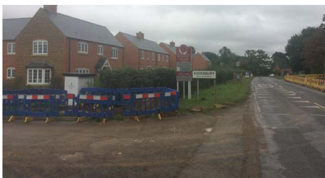
Development on Milton Road on approach to Adderbury
