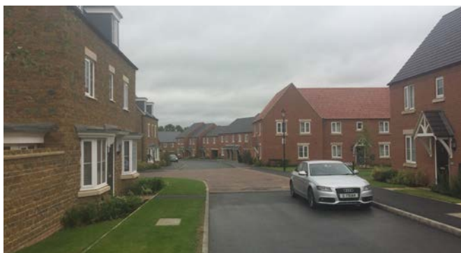
Example of new dwellings in the south-west of Adderbury
