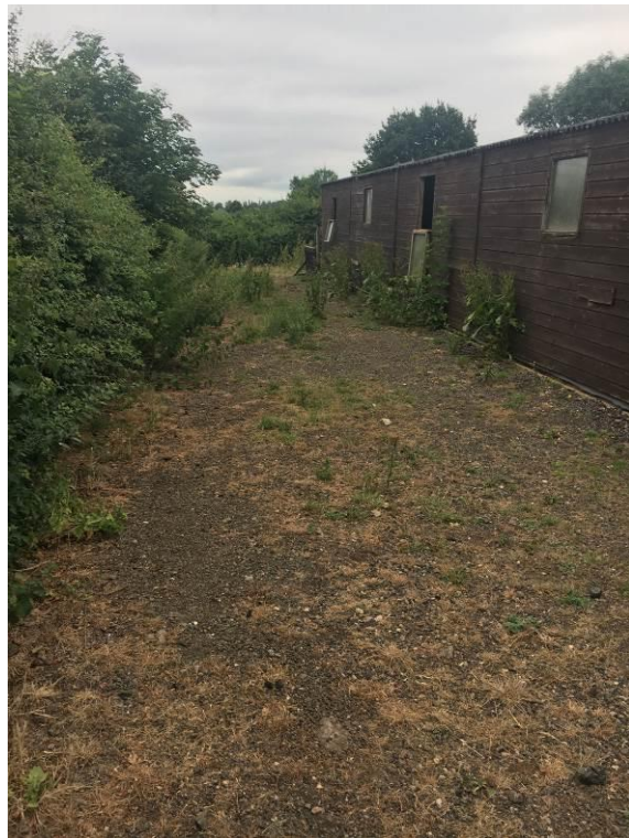
Localised Made Ground surrounding the stable area.
