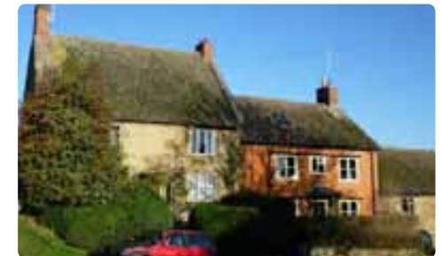
14 The Cottage (red brick dwelling)
