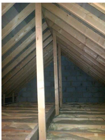
Plate 2: Internal view of the first roof void.
