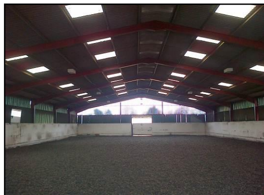
Plate 4: Internal view of B3
