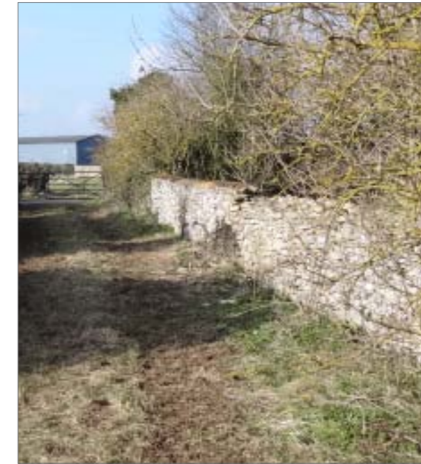
▲ Existing stone walls on site
