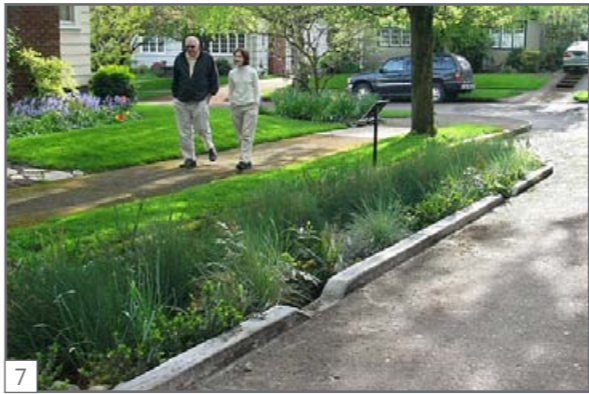
7 Swale Corridor Along Road Verge
