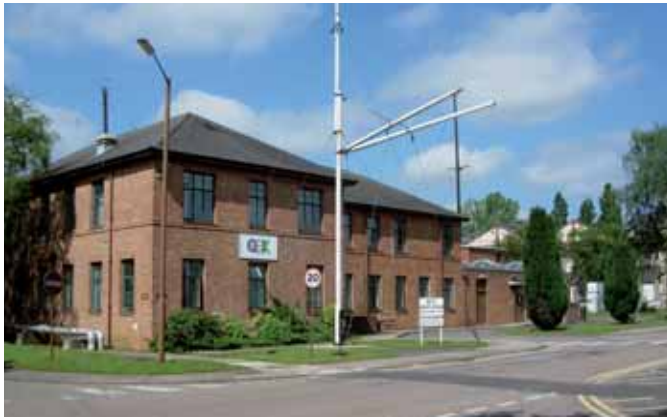
fig. 2.27 The 1920s buildings were constructed in traditional forms and materials (brick, slate) - office block No. 125
