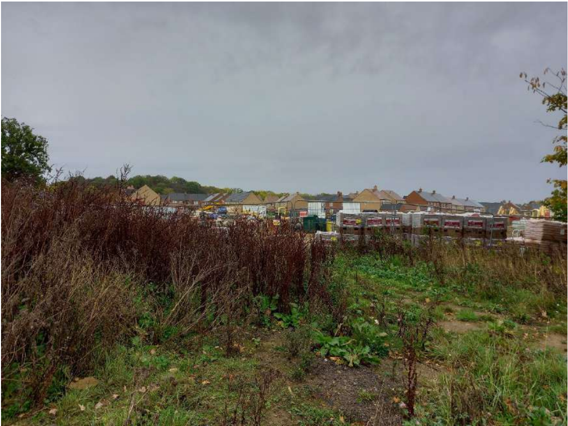
Image EDP 2.3: View of the adjacent residential development (Phase 1) under construction.
