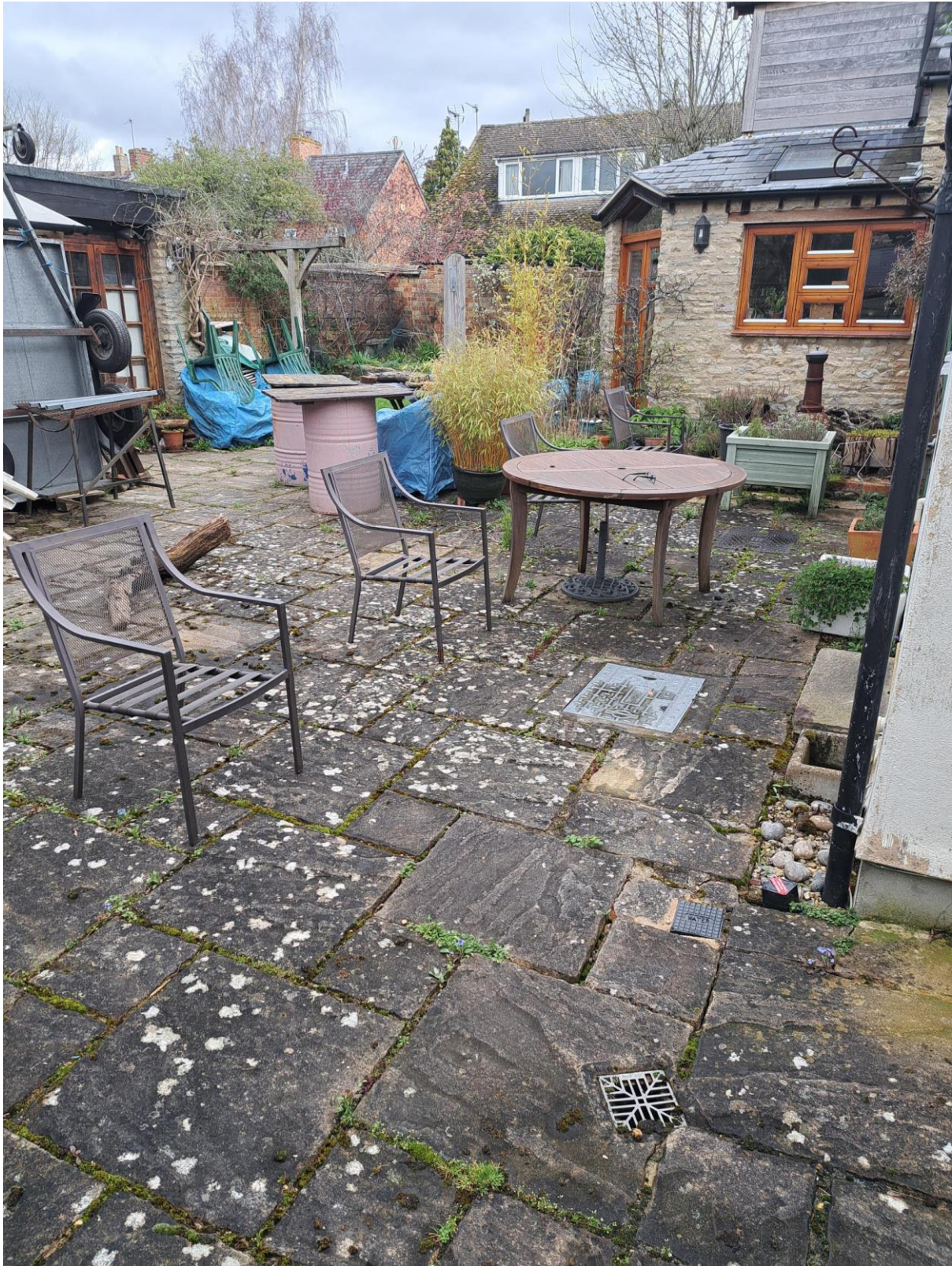
This is a view facing north. The western double gate/fence will run north/south on a line just to the left of the chairs shown in the picture. The northern gate will be installed behind the furthest chair shown in the photograph.
