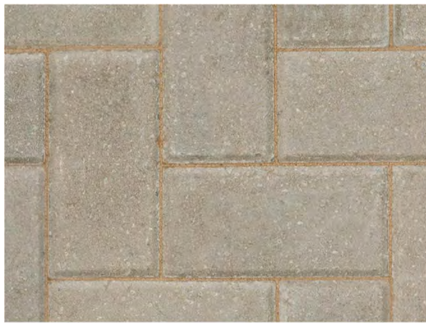
03 BLOCK PAVING TO CAR PARK CIRCULATION 020 natural
