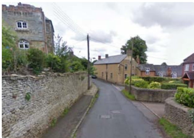
23. Wiring cuts through the view of the historic properties at the junction
