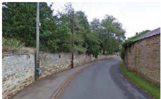
14. Walls are a characteristic feature in the village and are worthy of protection
