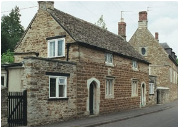
12. The Grade II listed almshouses, showing the difference between traditional and late 20th century windows
