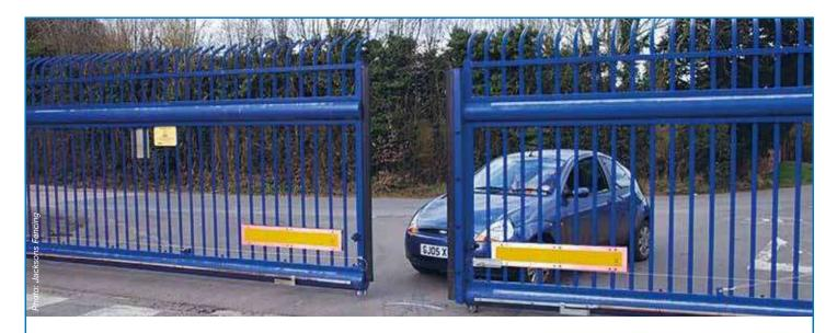
is to prevent a vehicle borne attack to penetrate a wall, door or window or to prevent parking of high sided vehicles close enough to the building to allow climbing to less secure windows or flat roofs.
