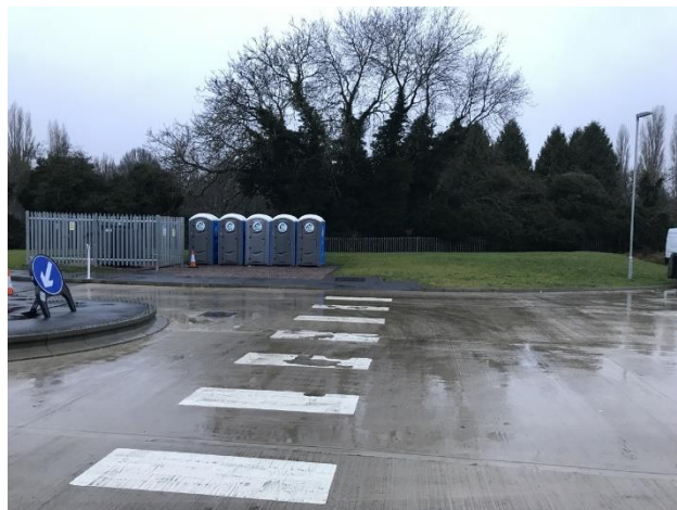
6. Site entrance with substation location.
