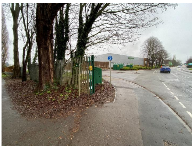
1.Existing Access into the site.
