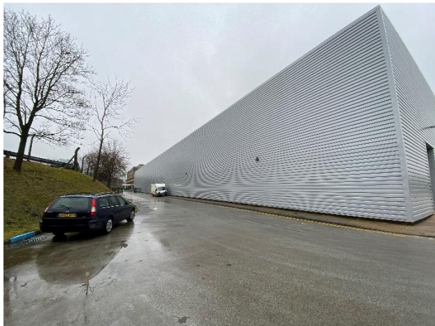
5. View of Western elevation with egress gate.
