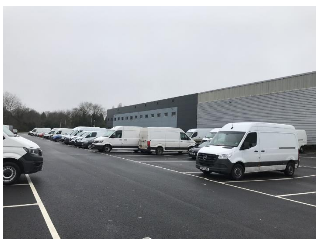
3.View of eastern elevation with existing car parking.
