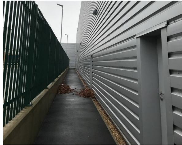
2. Rear of site with boundary fencing
