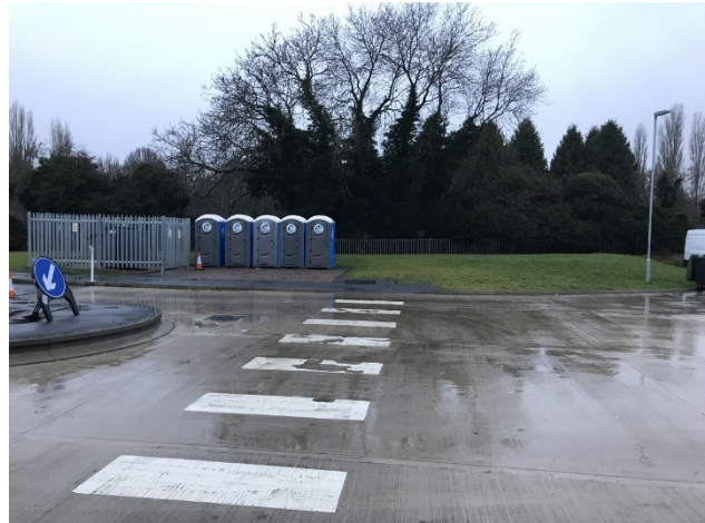
6. Site entrance with substation location.
