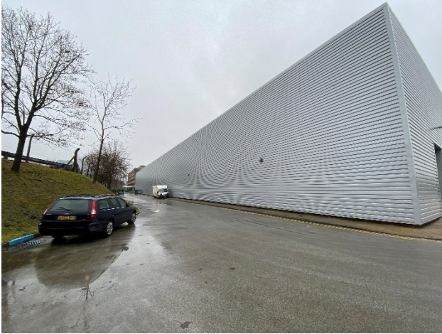
5. View of Western elevation with egress gate.
