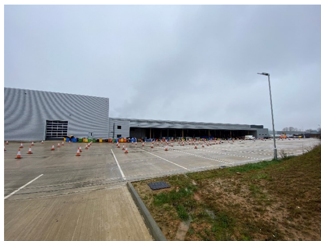
4. View of south elevation with loading docks and existing parking.
