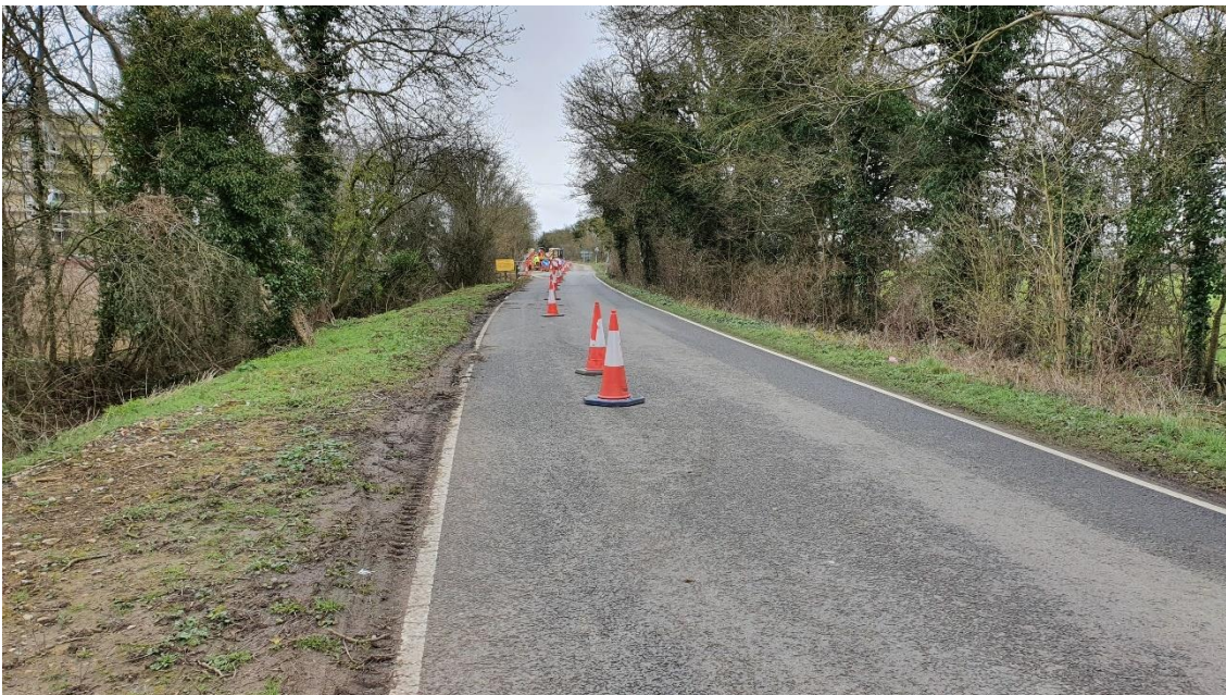
Figure 1: Existing ditch on western side of Wendlebury Road.
