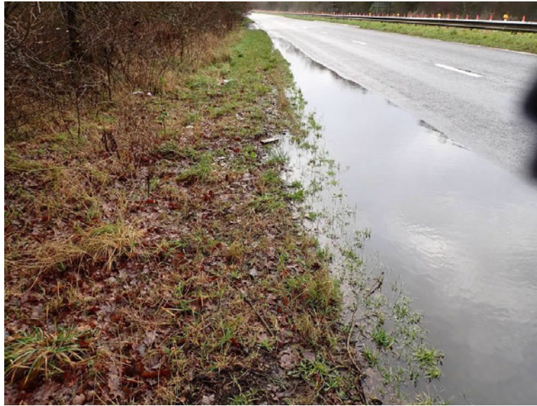
Pooled water on Frieze Way flowing over verge and directly into Triangle ditch at point in centre of photo on 02.01.2024 after very heavy rainfall. Photo J A Webb.
