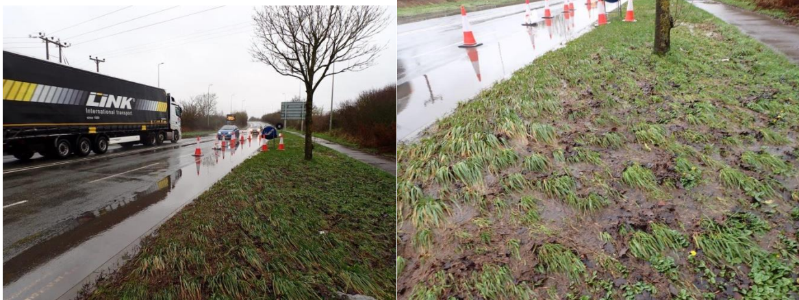
02.01.2024 Oxford Road next to Triangle partially flooded after very heavy rain, evidence of flood flow over verge (grass leaves direction) and footpath into the Triangle on east side. Photo J A Webb.
