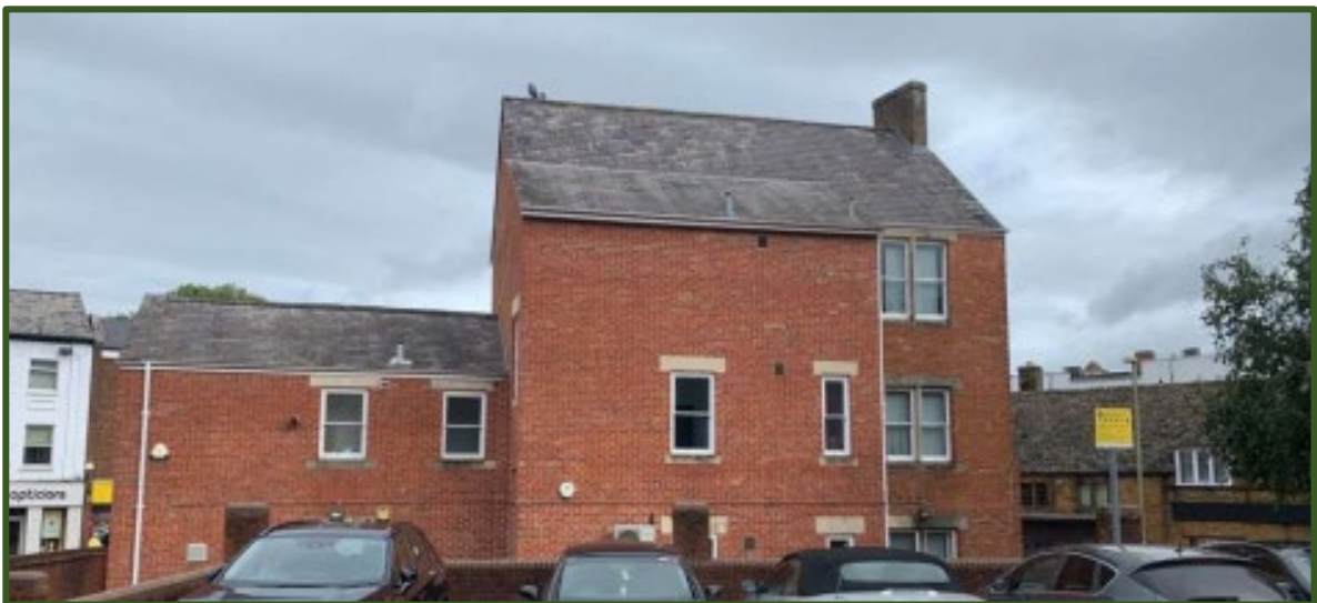
Photograph 5. Commercial premises in north of site
