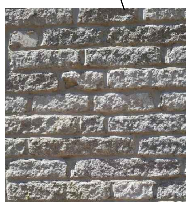
STONE AND MORTAR SAMPLE TAKEN FROM THE EXISTING HOTEL TO BE USED
