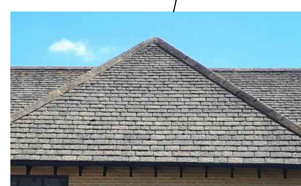
TILE SAMPLE TAKEN FROM THE EXISTING HOTEL TO BE USED
