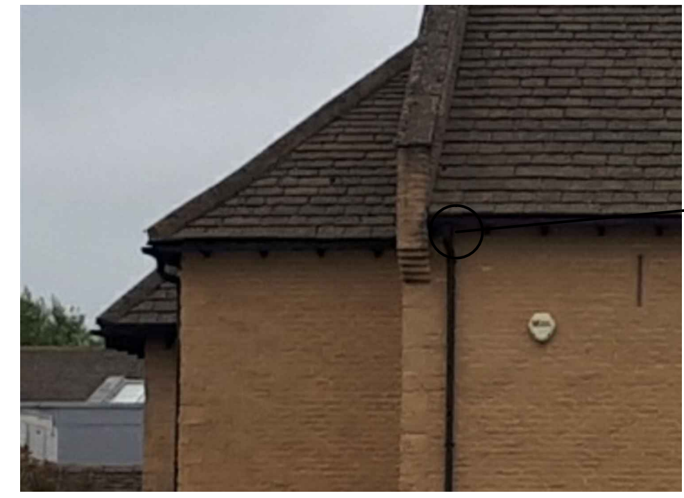
TYPICAL CAST IRON BLACK RAIN WATER GOODS TO BE USED TO MATCH MAIN HOTEL
