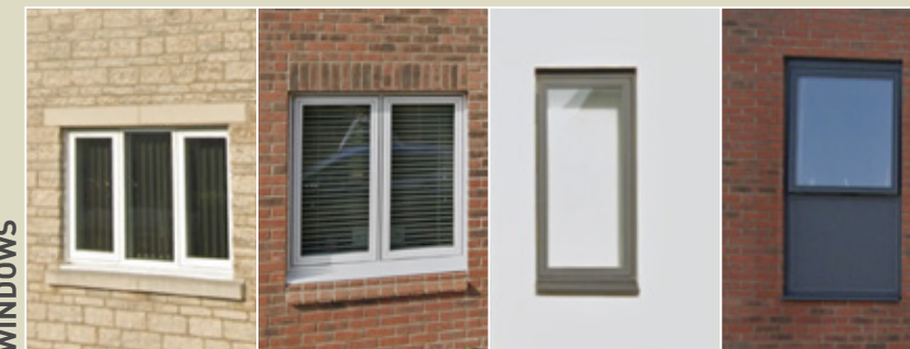
Stone header and cills. Brick header and brick cills. Contemporary style with no header or cills.
