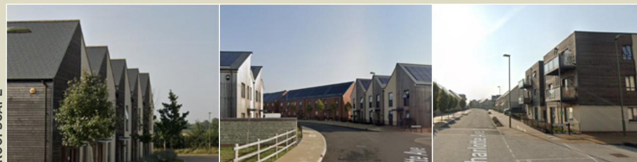
Strong rhythm and uniformity to the roofscape is common within the development to form signature frontages. Roofs are orientated (wherever feasible) to maximise efficiency for PV solar panels. Generally simple pitched roofs with no evidence of dormers or chimneys. Flat roofs to apartment buildings.
