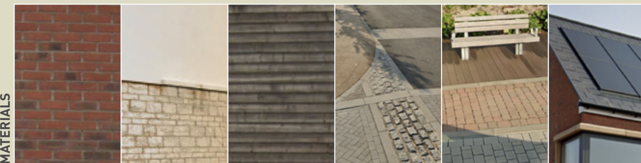
Walls: Varied use of stone; red bricks; white/cream smooth render and wooden cladding. Public realm: Varied hard landscape materials and street furniture to separate uses and hierarchy. Roof: Predominantly grey slate with PV solar panels.
