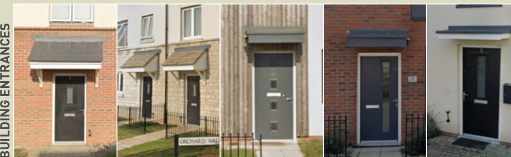
Pitched door canopies to the traditional style dwellings. Flat door canopies to more contemporary house types.
